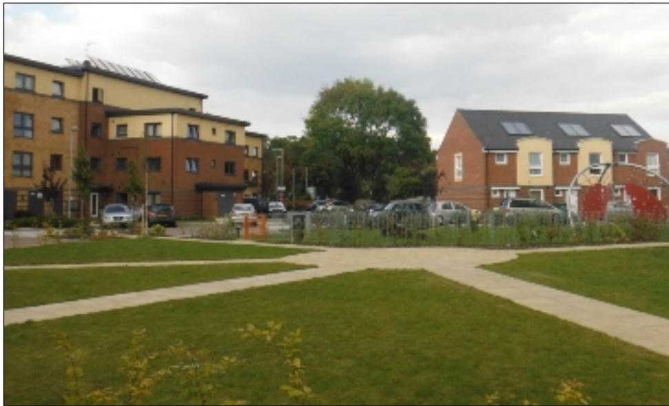
Figure 9-1: Former Fire & Ambulance Station development, Whippendell Road
